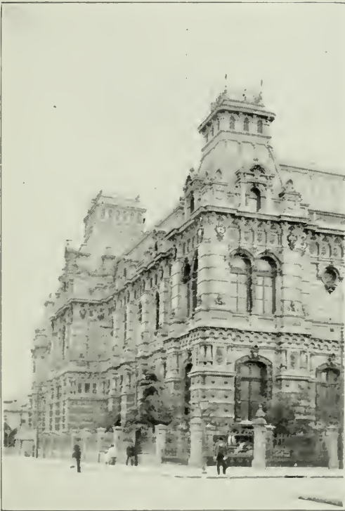
THE CITY WATER RESERVOIR OF BUENOS AIRES, ITS WIN- DOWS ARE "MAKE BE- LIEVE," NOT REAL.
